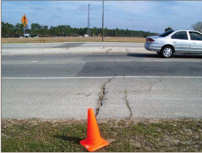
Figure 3. Willow Creek fault scarp across Highway 249. Note the several fractures and asphalt patches on the road. The picture was taken facing east. The car was going toward the bridge on the south (upthrown) side of the fault.
